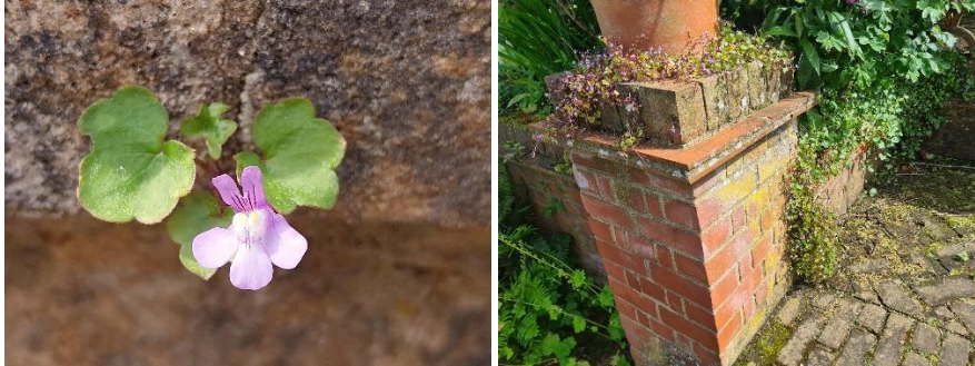
Photos by David Cooling (left) and Julie Bunker (right)
